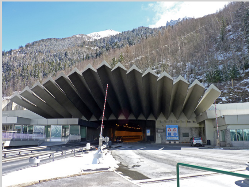
Exit portal - French side
