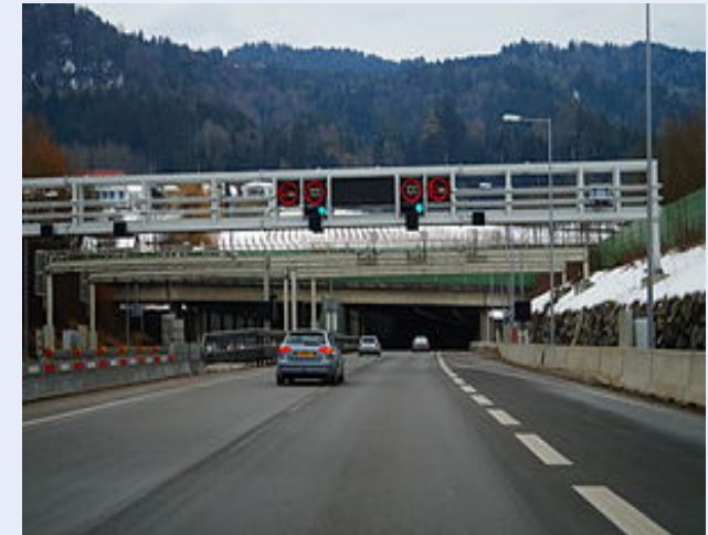
Tunnel in Austria
