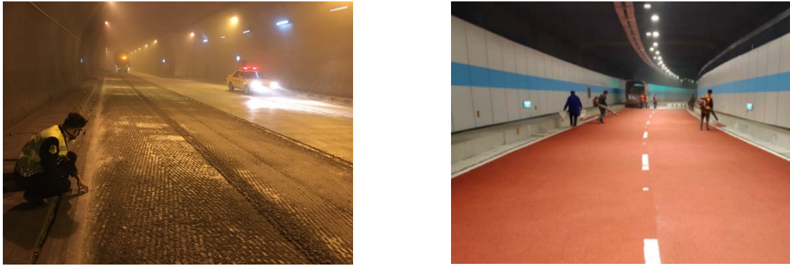
Figure11: Anti-sliding performance of pavement in tunnel
