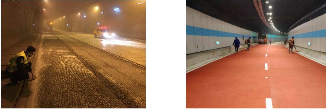
Figure11: Anti-sliding performance of pavement in tunnel
