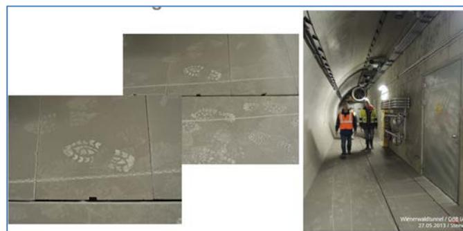
**Figure 3:** Dust load in a cross passage of the Wienerwald Railway Tunnel / ÖBB Westline
