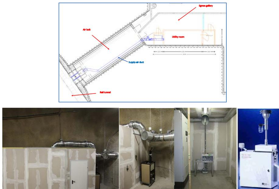
**Figure 4:** Test room within the Unterwald evacuation gallery – layout (above); utility room (left); PM measurement devices / TEOM, Sharp & PARTISOL (right)
