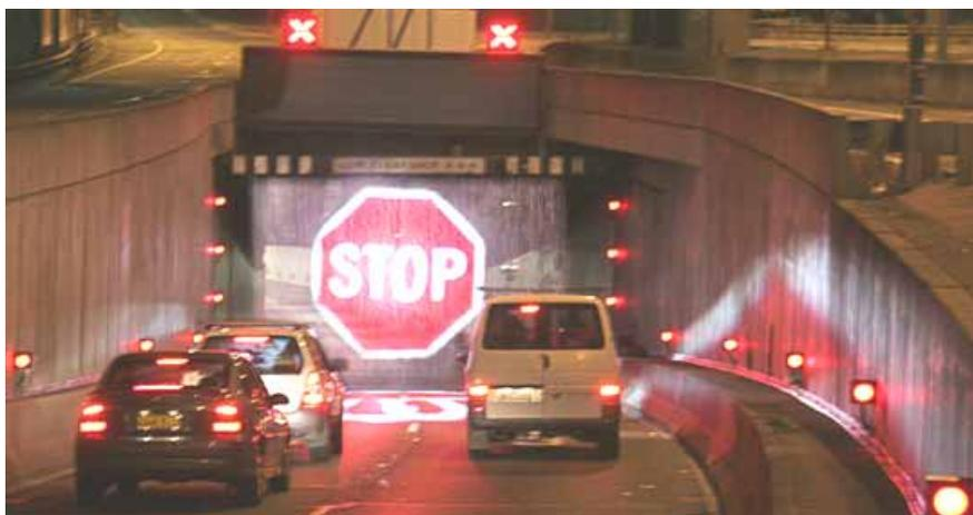
**Figure 3:** The “Softstop” system being used at the portal of Sydney Harbour Tunnel
