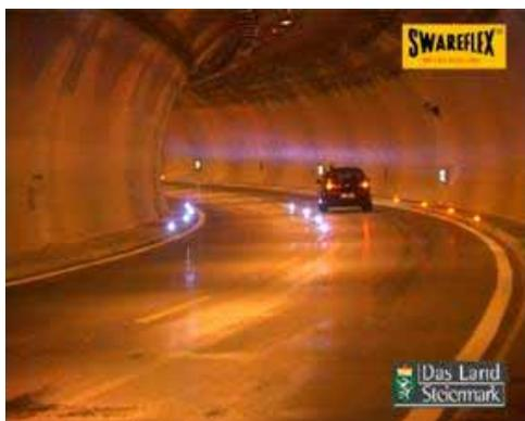
in the Assingberg tunnel. Tests showed that a four unit light sequence might be beneficial. Apart from its impact on traffic speed, such an intelligent LED lighting system has the further advantage that it provides for active sequencing of exit indicators as well as the possibility to activate centre line indicators.
