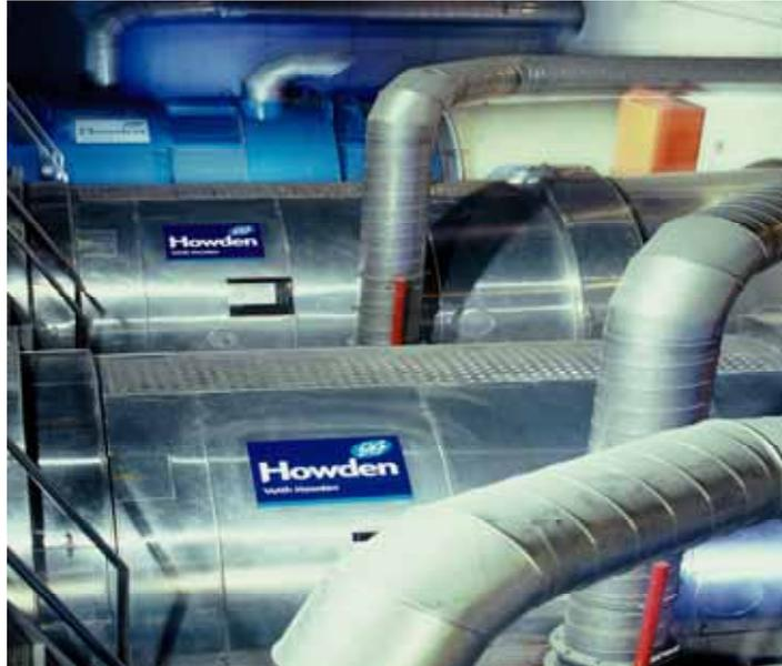
**Figure 1:** Typical installation of axial flow fans in parallel operation
