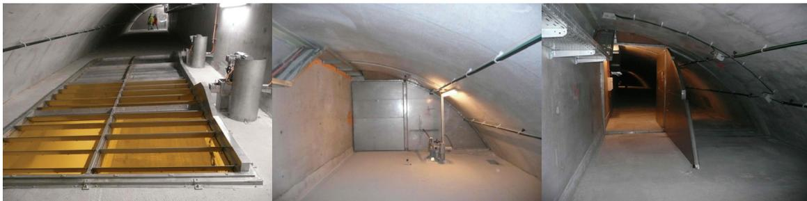
**Figure 6:** Fresh-air injection device: damper (left), blocking element closed (centre), blocking element open (right); construction IWN GmbH
