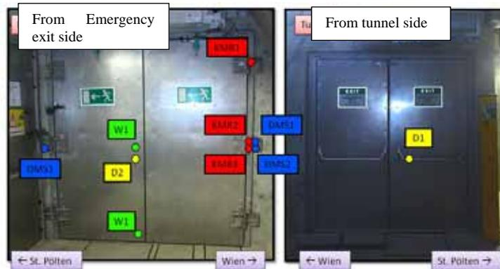
**Figure 2:** Arrangement of the sensors in the Wienerwaldtunnel [3]
