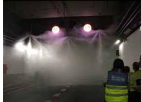
**Figure 2:** Water mist system in the M30 tunnels
