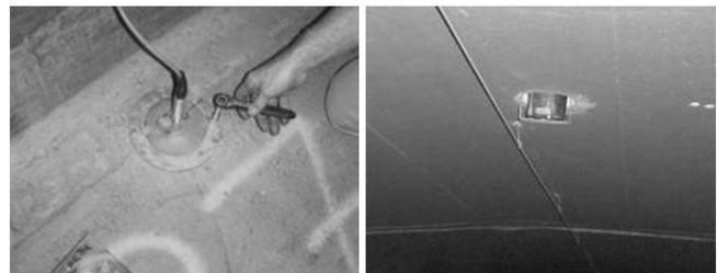
FireGuard installation: view from top of the intermediate ceiling (left) and under the intermediate ceiling (right). Also visible is the linear heat detector
