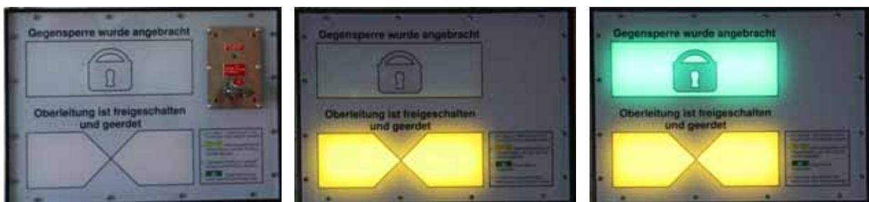
control panel - catenary system not disconnected and not grounded, and also not secured against reconnection
