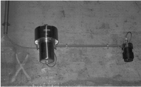
Test installation: VisGuard (left) & FireGuard (right)
