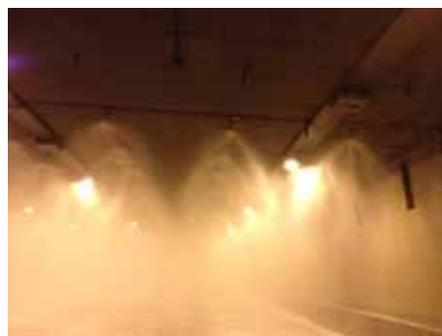
**Figure 1:** Deluge system in the Mount Baker tunnel
