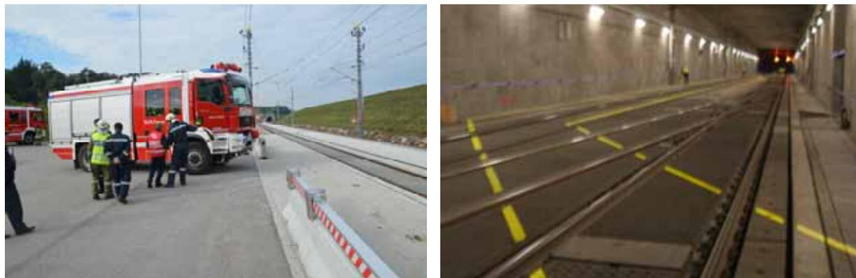
**Figure 3:** Railway tunnel accessible for rubber-tired vehicles
