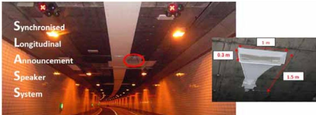
**Figure 1:** Illustration from [13] of SLASS loudspeaker system in the Elbe tunnel.
